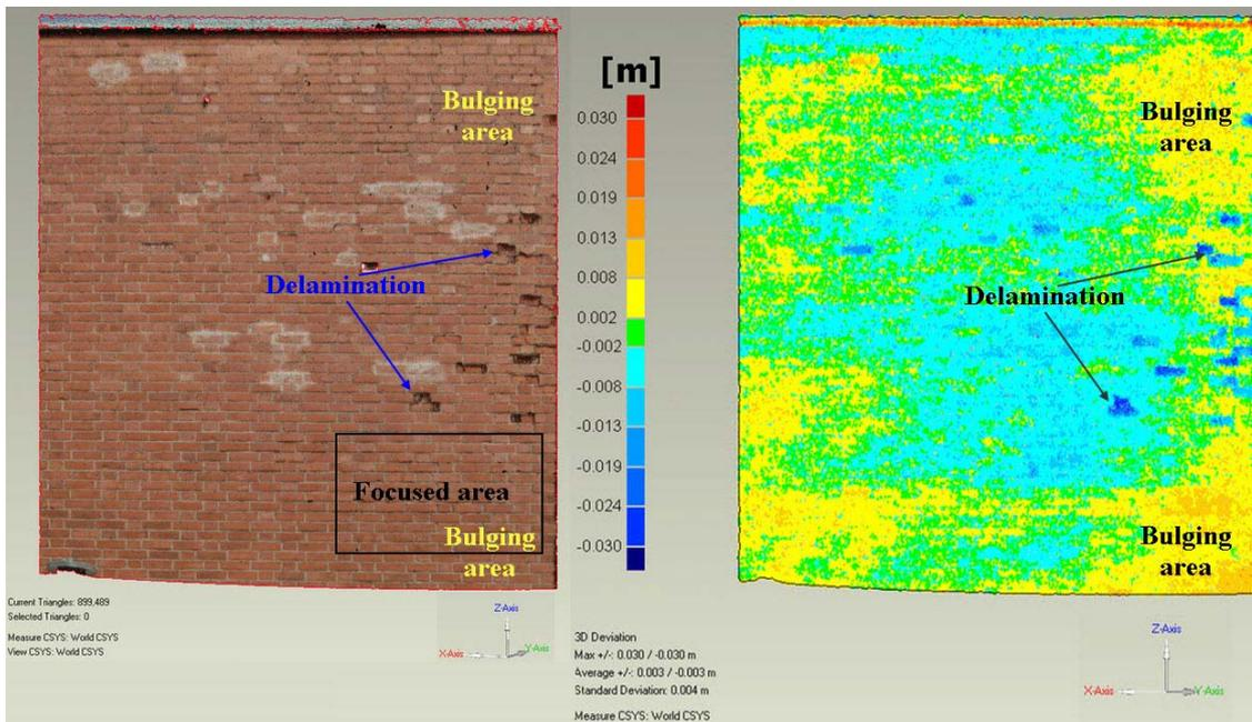
Figure 13. Delamination of bricks and the deterioration of joints detected from the laser scanning data.
